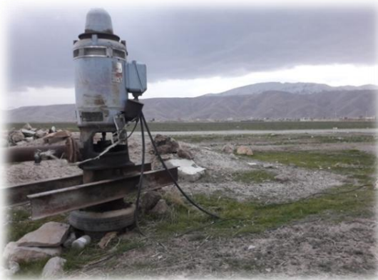
Fig. 8- Khanmirza plain, north-eastern of Dehsahra UTM Coordinates= x: 510956 - y: 3487132 Well piping: about 40 cm (18/08/2022)
